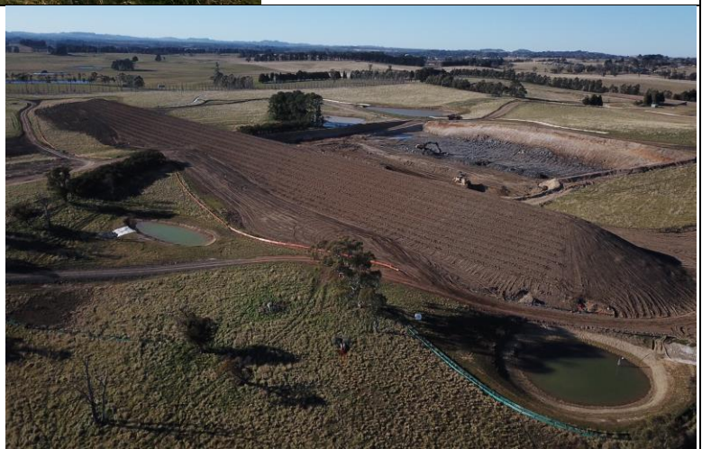
Plate 4 Central Visibility Barrier – Soil Spreading Complete with Rip Lines for Tree Planting Source: Austral Bricks Date: August 2021
