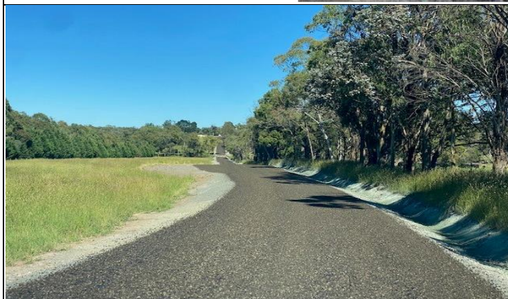
Plate 7 Sealed Quarry Access Road with Passing Bay and Hydromulched Drain Source: Austral Bricks Date: December 2021
