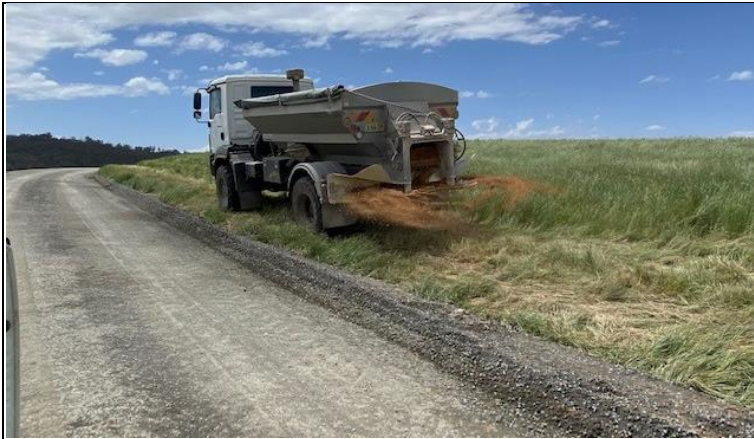
Plate 1 Spreading Gypsum Prior to Soil Stripping – Western Access Road Drain Source: Austral Bricks Date: November 2021
